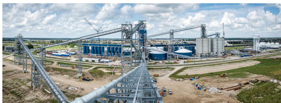
Louis Dreyfus Commodities LLC's flagship Mississippi River export facility at the Port of Greater Baton Rouge features a grain elevator capable of annually handling as many as 5 million metric tons of grains and oilseeds.
